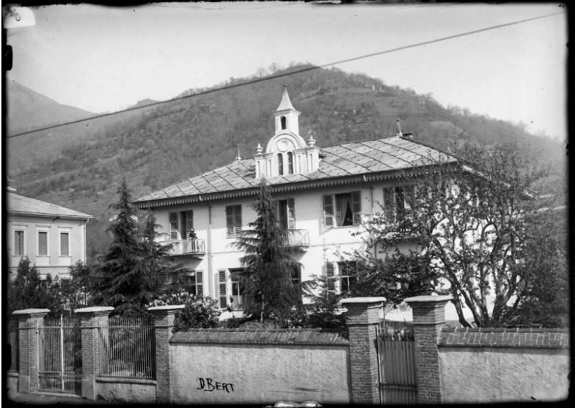
Torre Pellice. Foresteria
